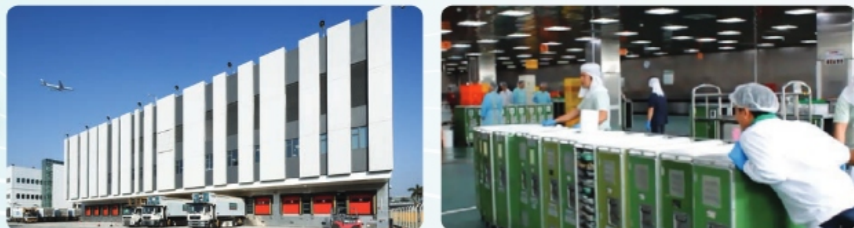
HONG KONG CATHAY PACIFIC CATERING SERVICES II
